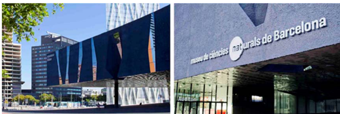
The Natural Science Museum of Barcelona, located at an outstanding building made by the Swiss architects Herzog & De Meuron for the Barcelona Forum in 2004.
